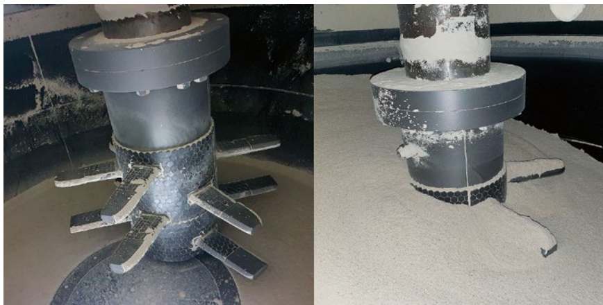
Figure 2 The mixing tool system after four years of operation, with and without material inside the mixer. (© Dörentrup Feuerfestprodukte)
